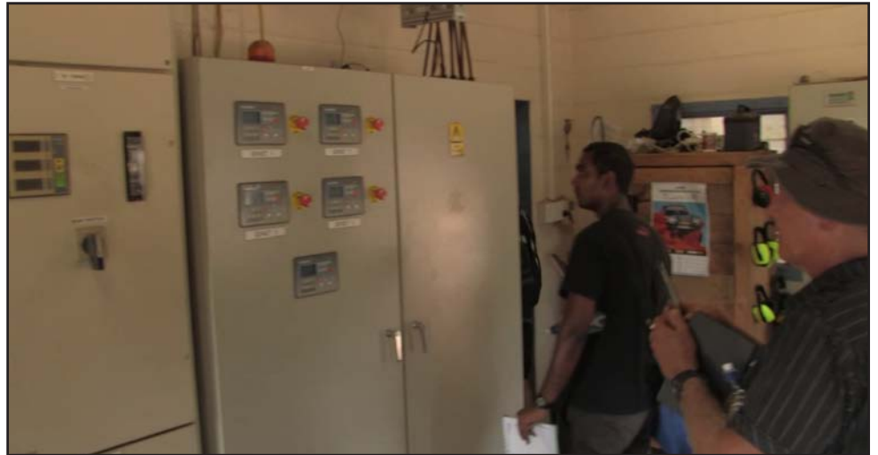
Keen bidders look at Mangaia Energy setup
